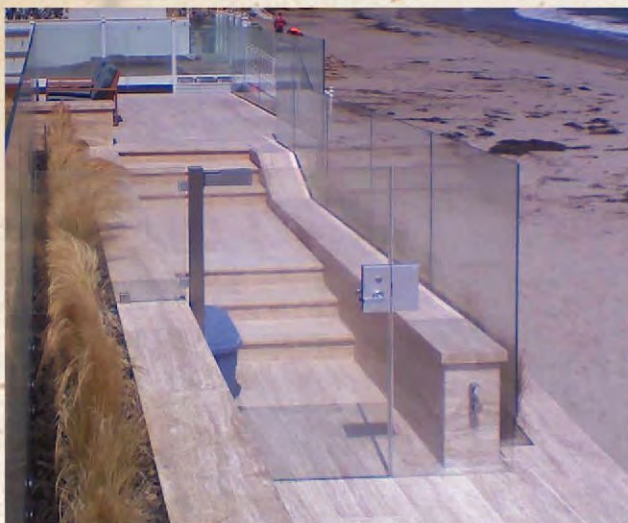
Custom Gate with custom centerlock/strike housing and Latchlock .
