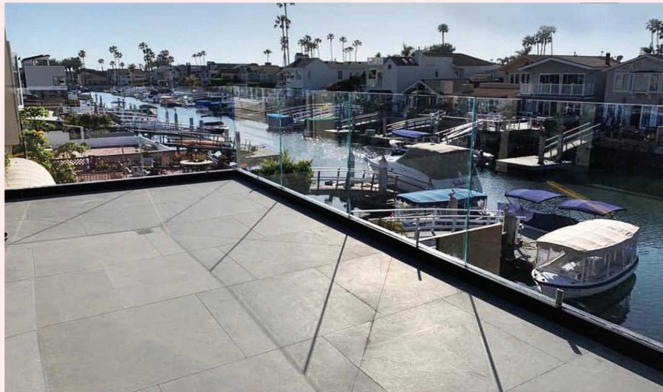
Bronzed Anodized Finish Rapid Dry-Set Guardrail System with Laminated SentryGlas®
