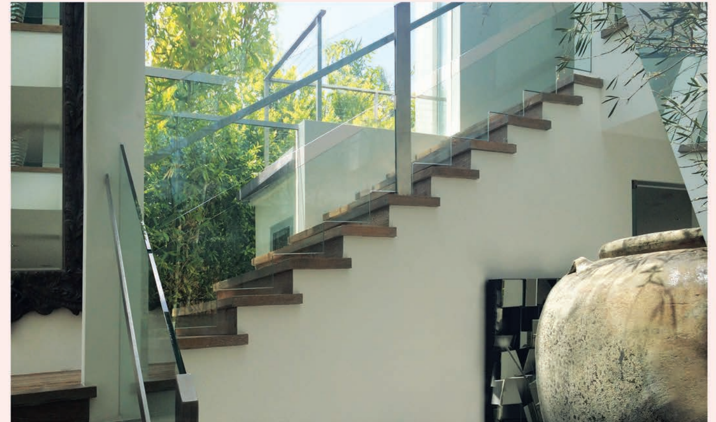
Custom Handrail System with Custom Cut Glass
