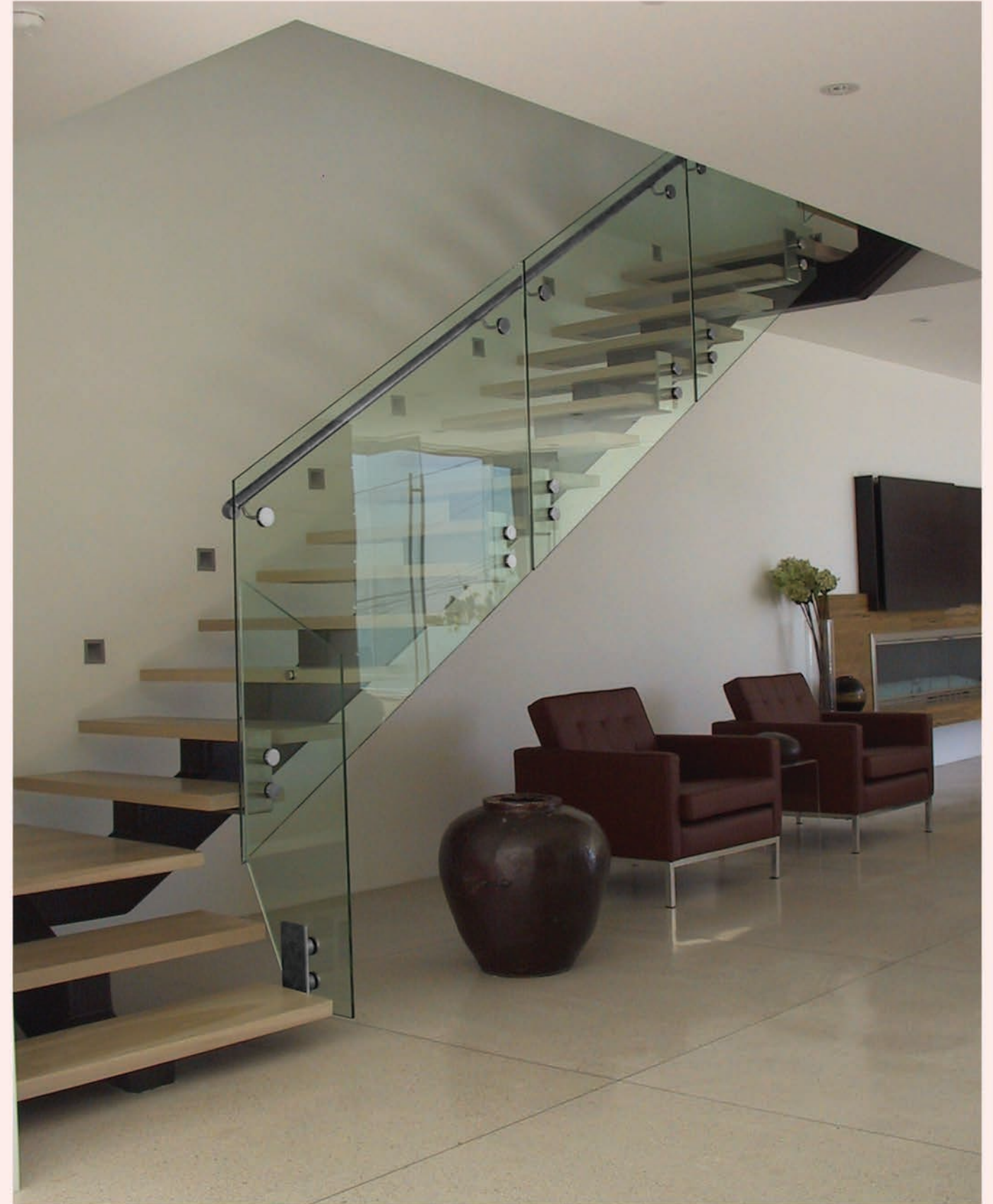
Elegante Handrail System with Square Stand-Off Mount Brackets and Laminated SentryGlas®
