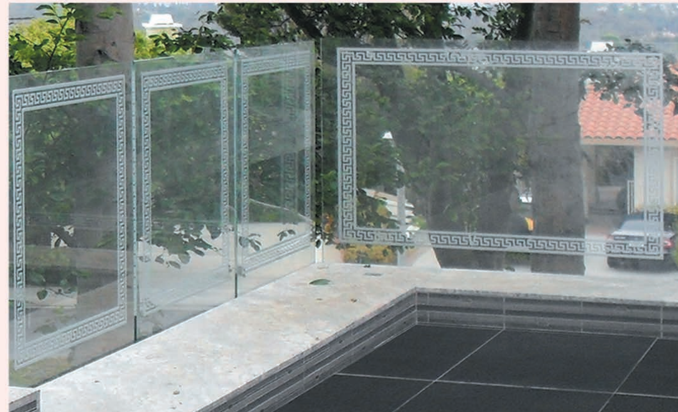
Traditional Guardrail System with Custom Design Sandblast Border
