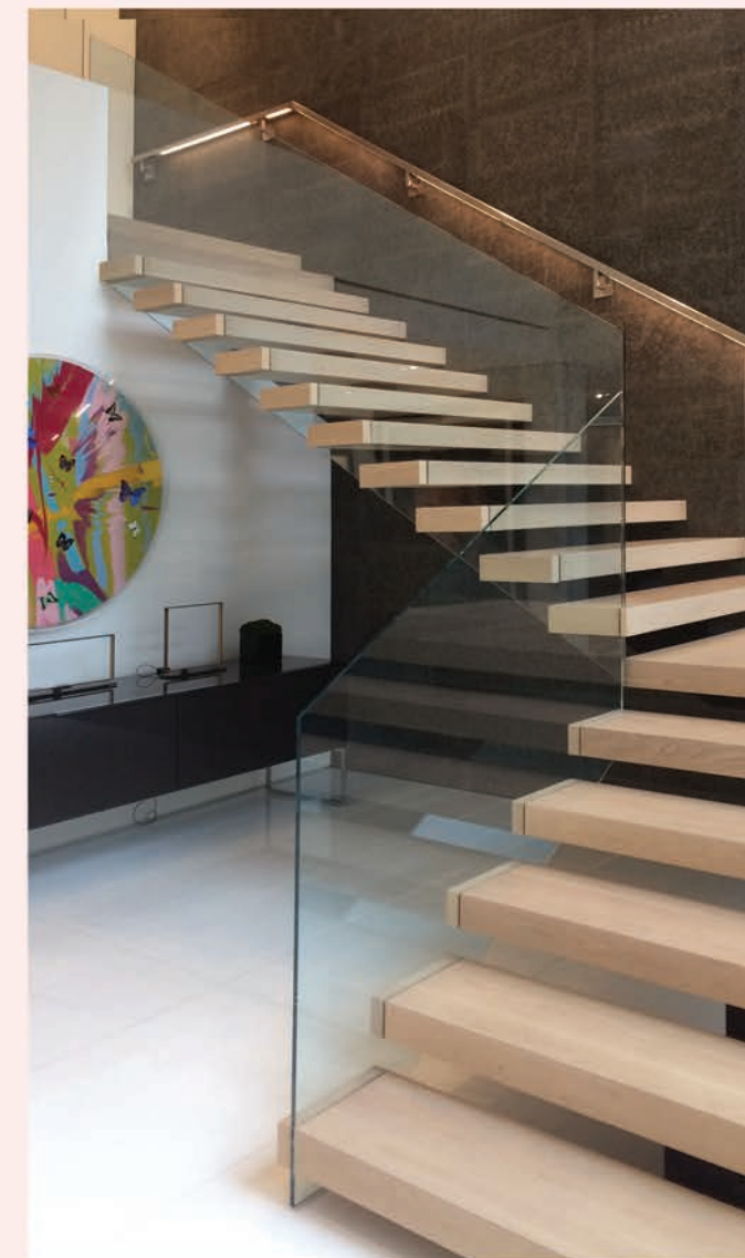
Handrail Glass Cut to Patterns with Custom Cut-out
