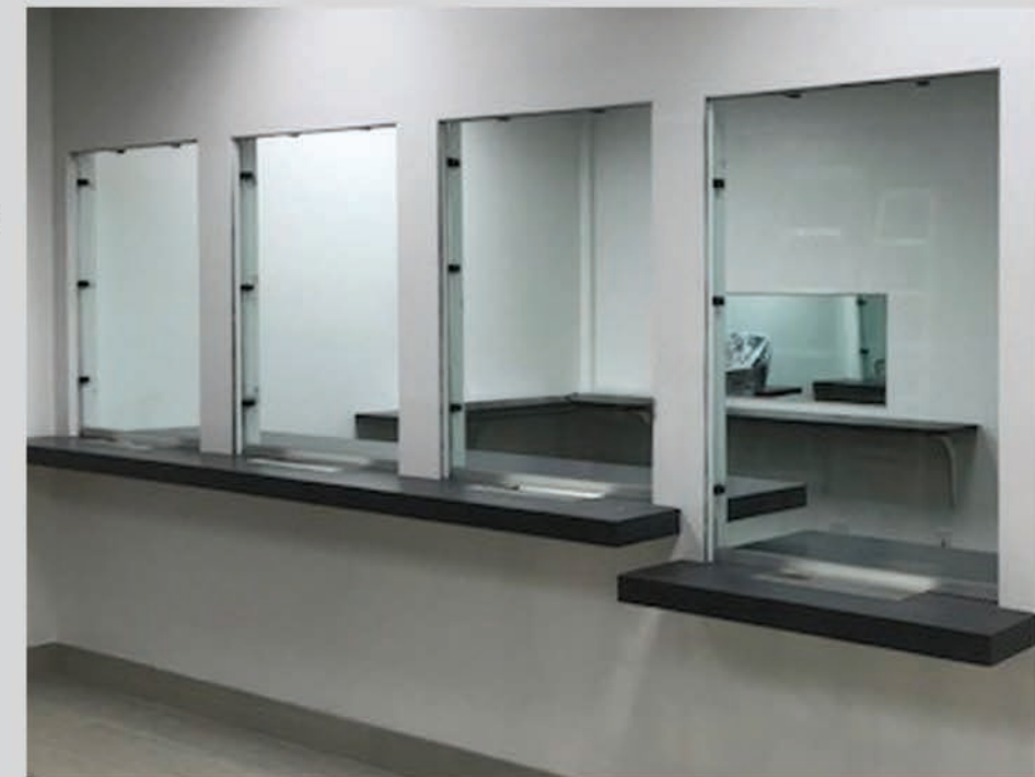
Transaction Windows with Level 1 Bullet Resistant
