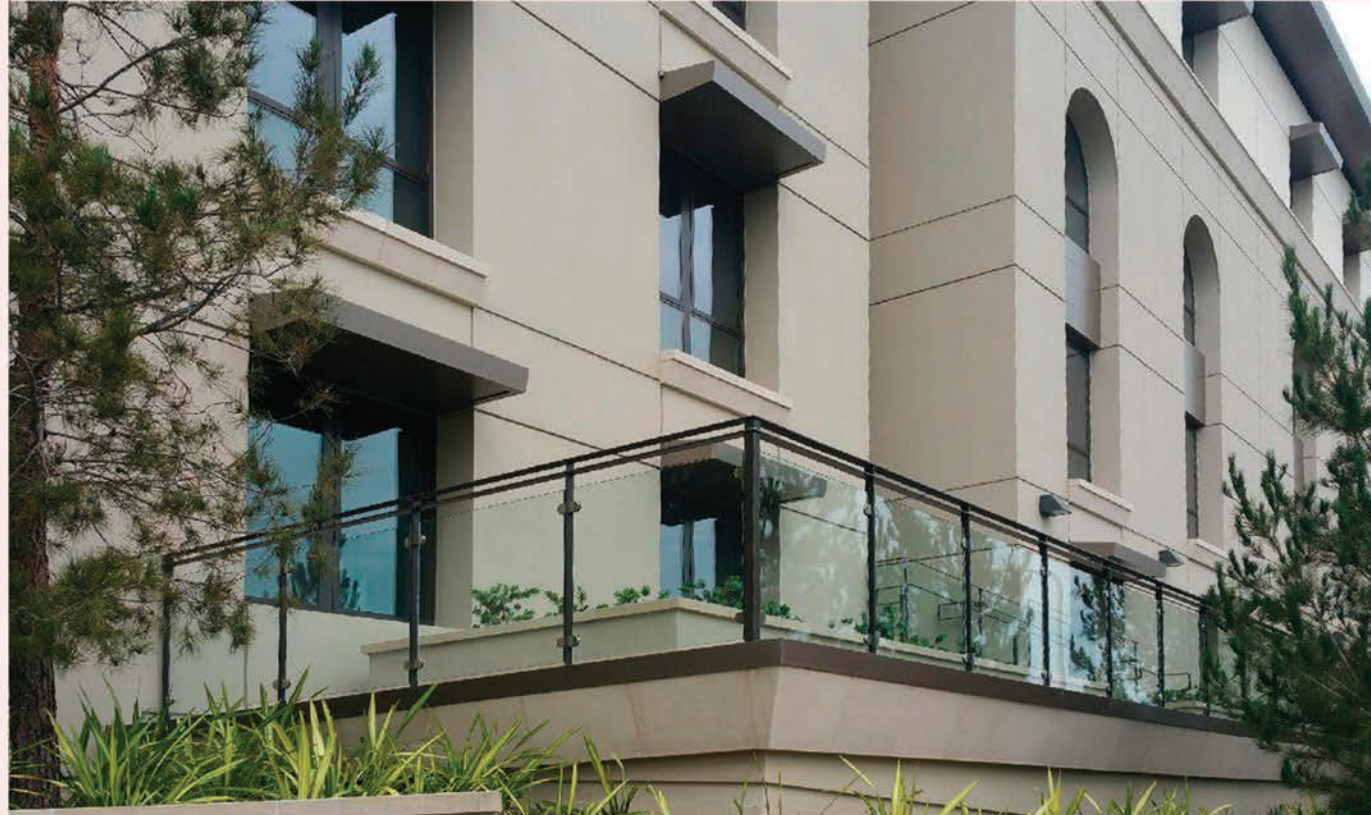
Guardrail with Custom Post in Bronzed Anodized
