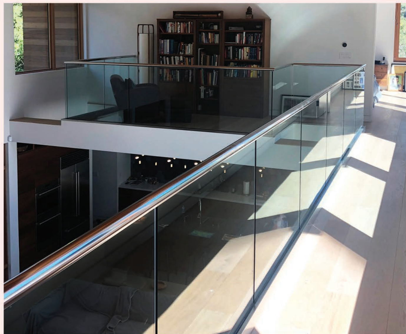
Traditional Handrail System with Round Brakeformed Top Caps in Polished Stainless Steel
