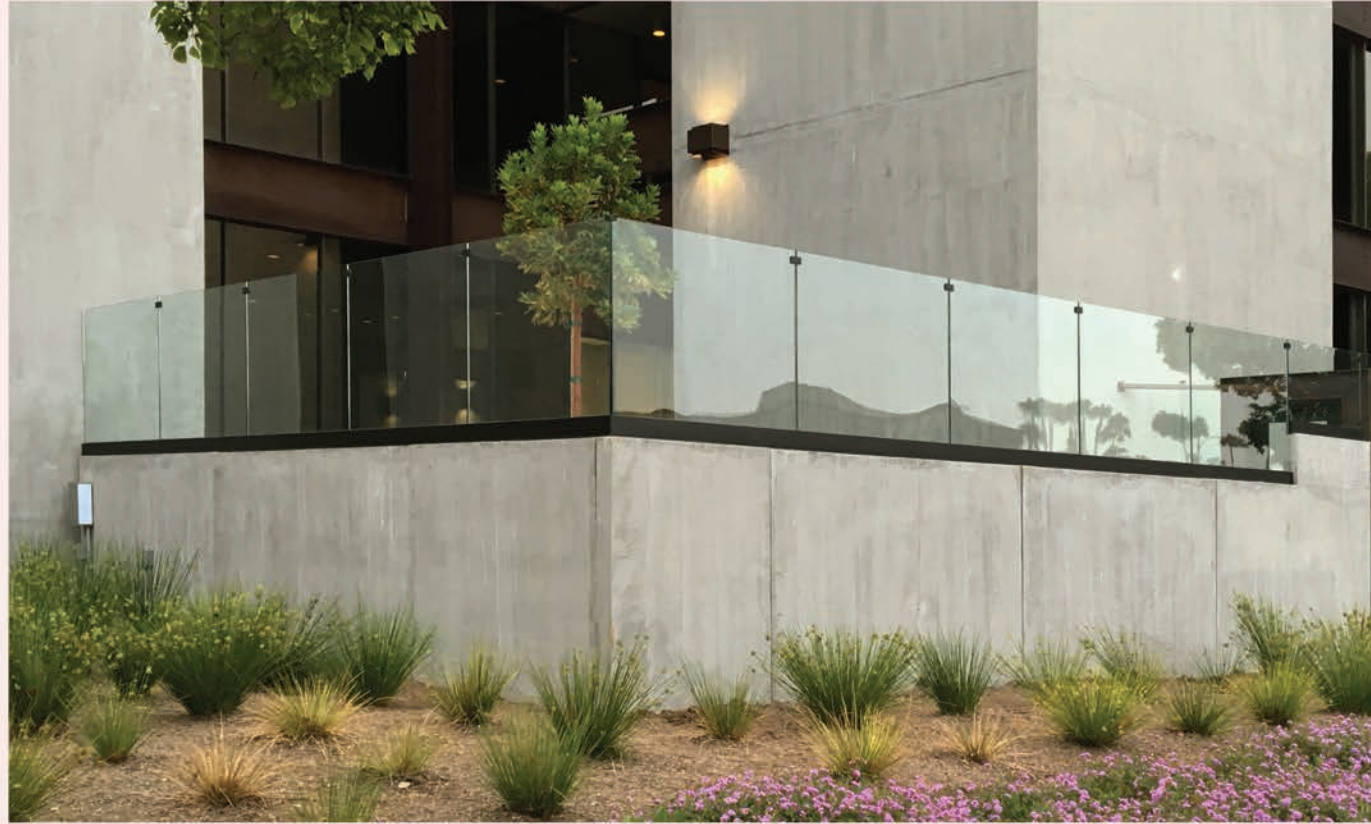
Dark Bronze Anodized Rapid Dry-Set Guardrail System with Laminated SentryGlas®
