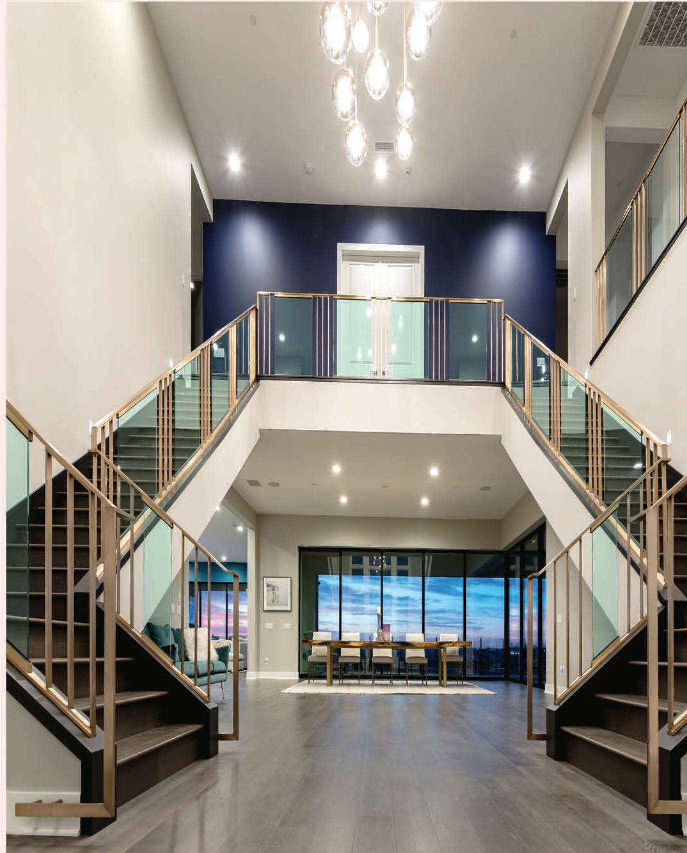
Custom Handrail System with Laminated Glass
