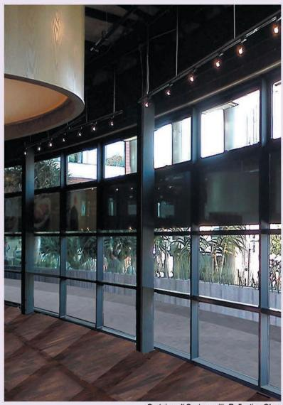
Curtainwall System with Reflective Glass
