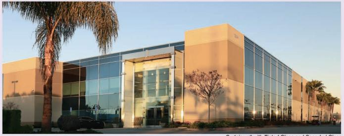
Curtainwall with Tinted Glass and Spandrel Glass
