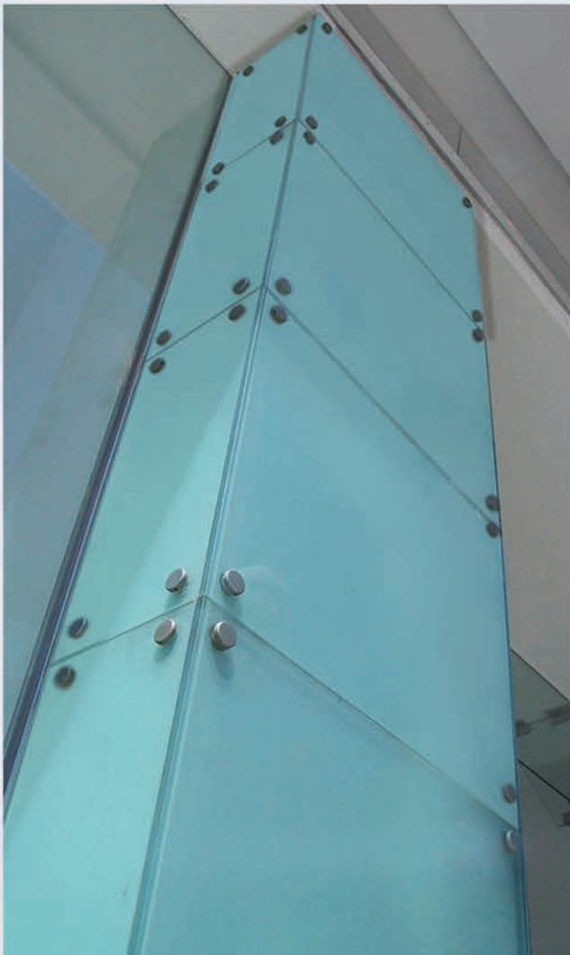
Spandrel Glass Panel Column Cover
