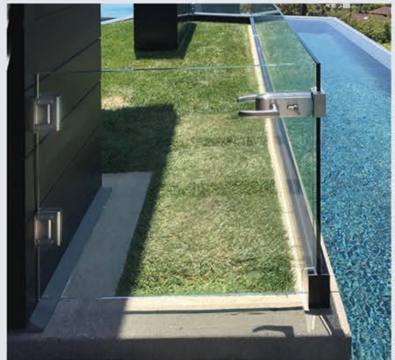
Security Gate with Custom Strike Application
