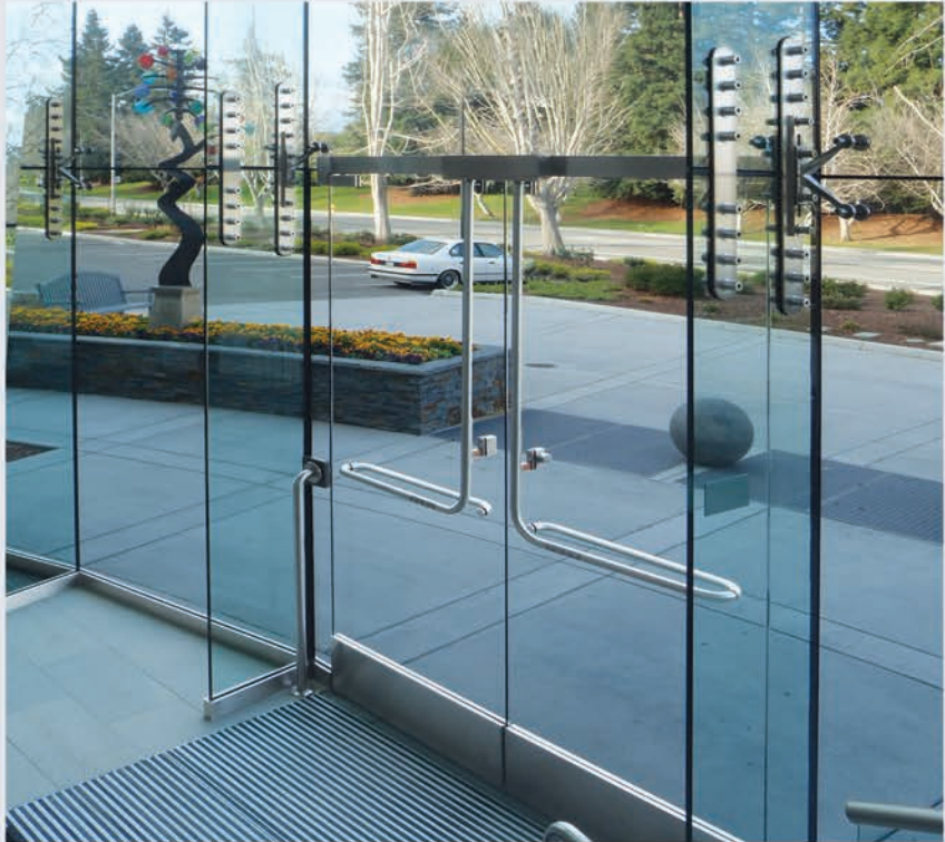
All Glass Entrance Doors with Laminated SentryGlas® and Panic Device
