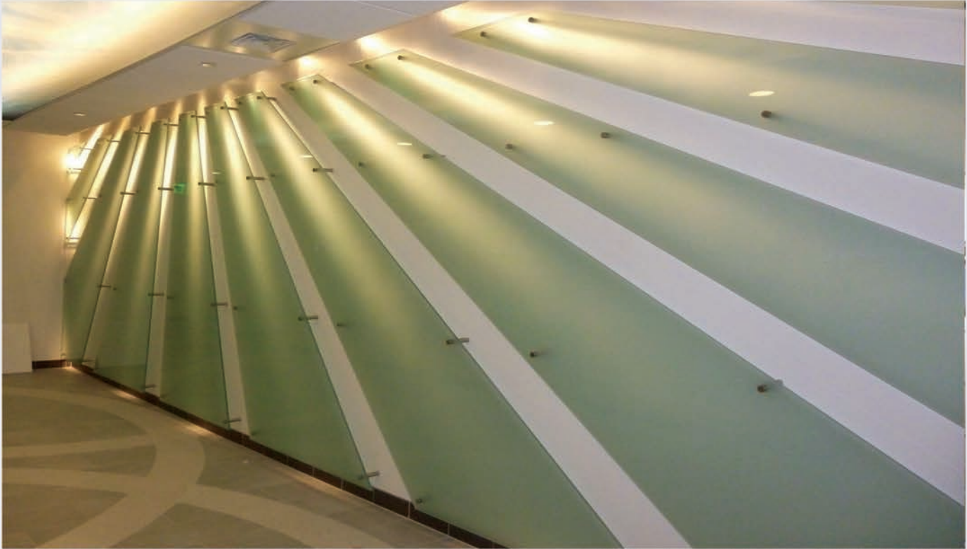
Infill Panels Glass Wall with Gradient Sandblast Design
