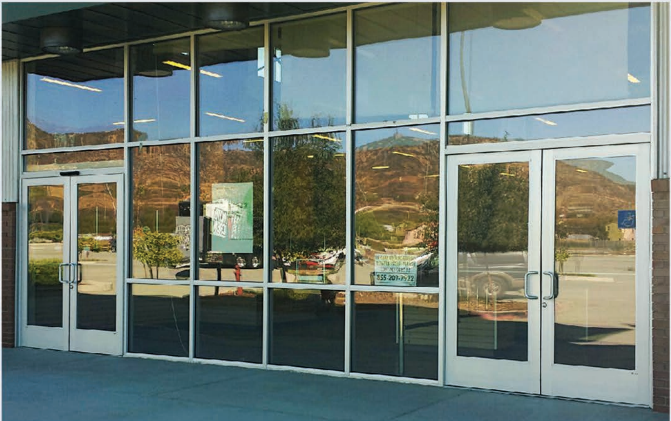
Complete Entrance System with PRL Fabricated Storefront , Doors & IG Units with Reflective Glass
