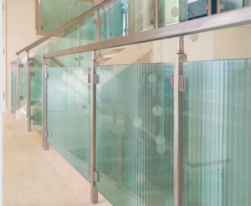
Laminated 1/4" Reeded Tempered 060 SGP/ 1/4" Clear Tempered Glass
