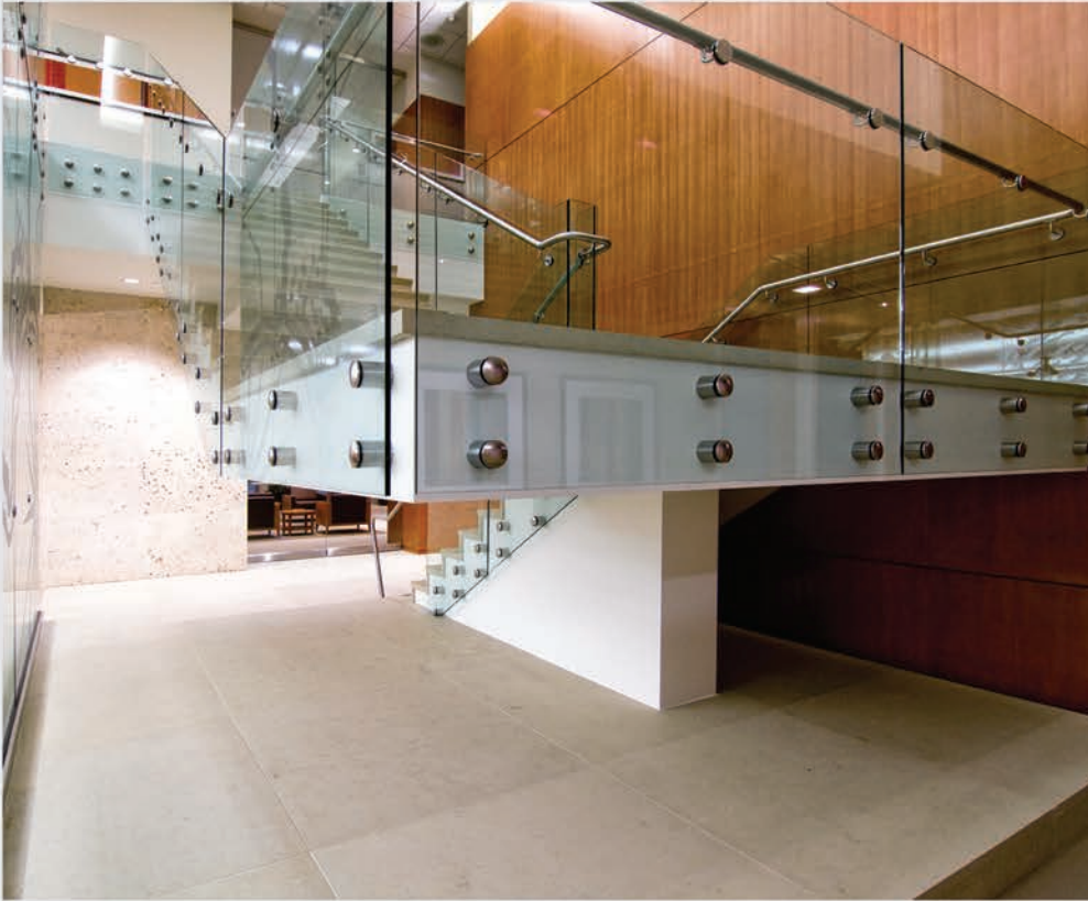
Elegante Stand Off System with Laminated SentryGlas®
