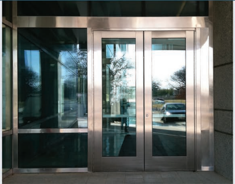
Full Frame Doors & Storefront Framing Clad in Stainless Steel
