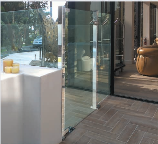
Security Access Gate
