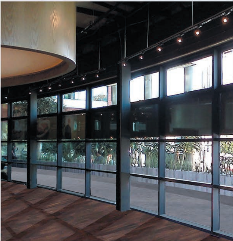
Curtainwall System with Reflective Glass
