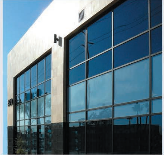
Curtainwall with Tinted & Spandrel Glass
